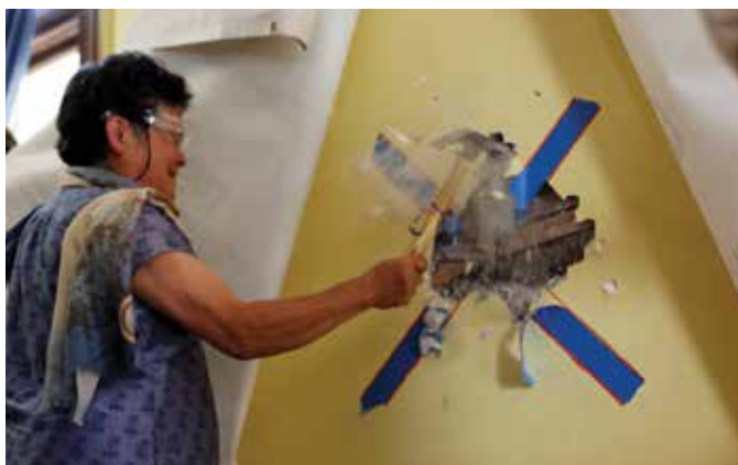
Li-Chiang Chu at the 2012 groundbreaking for the Sherman Hall Seismic Retrofit.
